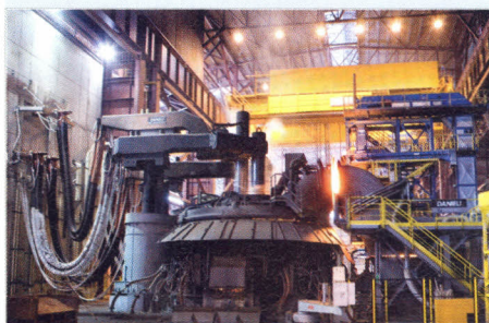
Typical Danarc EAF in operation
