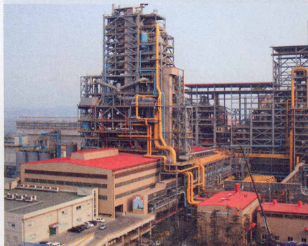
Existing No. 2 Finex ironmaking plant at Posco, Korea
