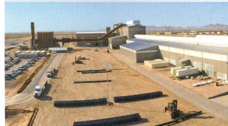
New micro-mill of CMC Steel Arizona
