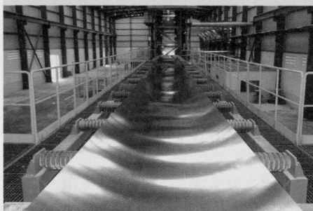
Exit section of a coating line
